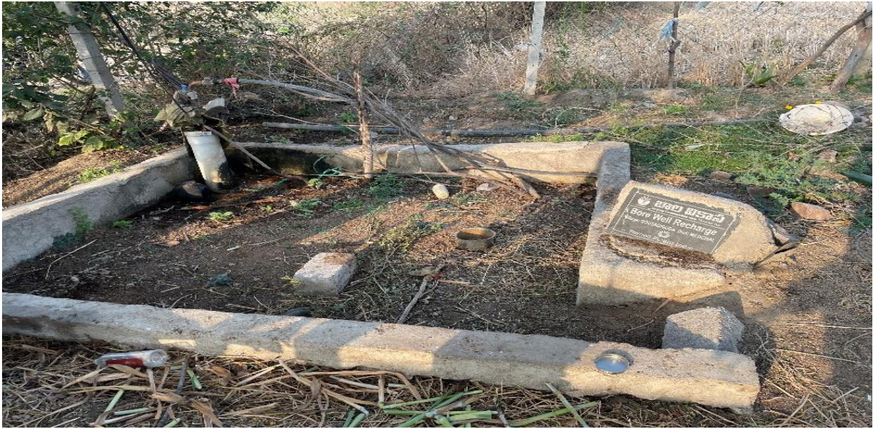
Figure 10: Constructed bore-well recharge pit with Pernod branding
